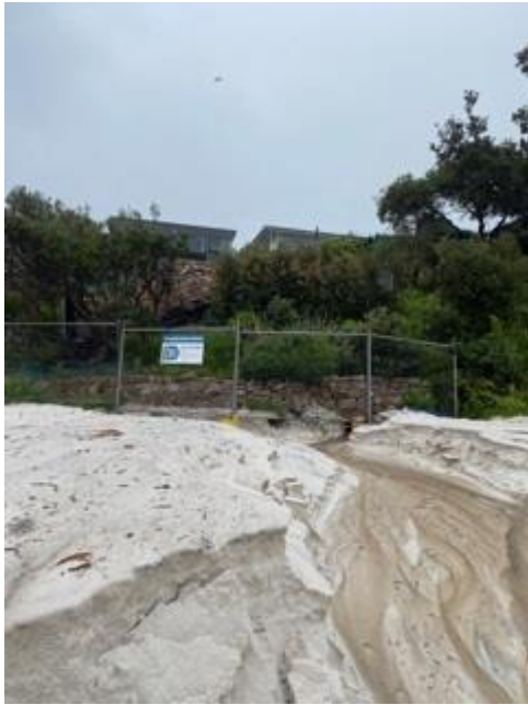
Figure 1: Storm damage, Seamans Beach, Hyams Beach January 2022
